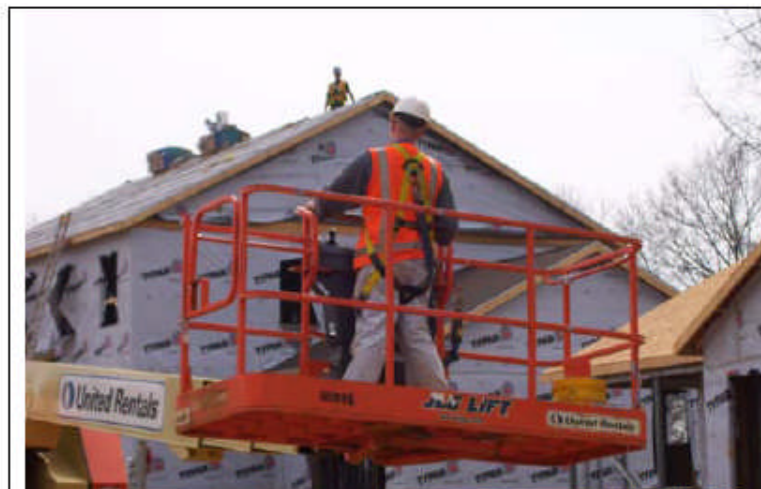
Figure 31 - Worker positioning an aerial lift.
