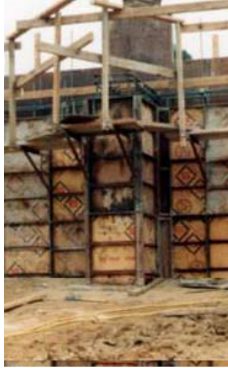
Figure 16 - A bracket-form scaffold attached to formwork.
