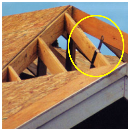
Figure 6 - A bolt-on anchor attached to a rafter.
